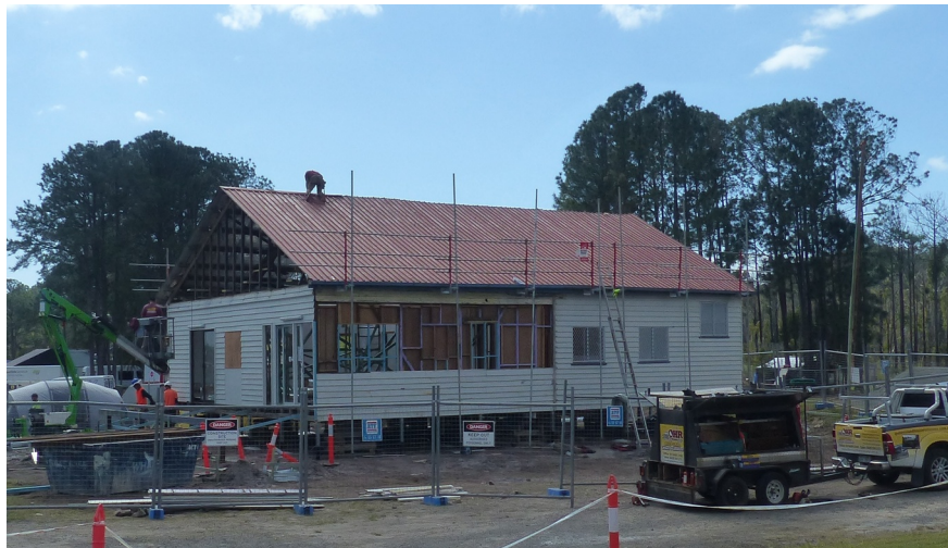
The Community Centre being assembled on our site – September 2018.
