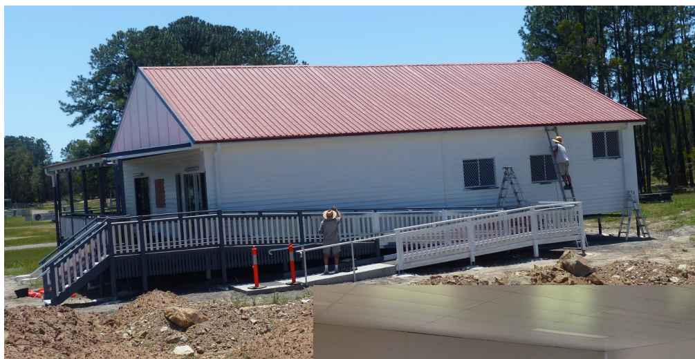
Work commences outside ....
